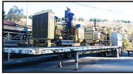
Port Gen Trailer , w/Two (2) Used Cat 3412 Generators, 545 KW, main breakers, w/ fuel tank, tandem axle ... P.O.R.
